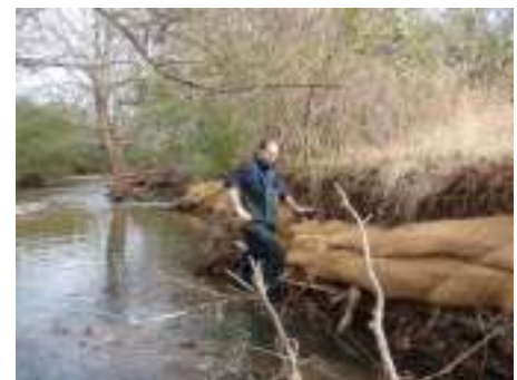
Kevin Burke inspects revetments along a stream in Spring Hill as part of the Duck River Opportunities Project. The Duck River is one of the most biologically diverse in the U.S. The revetments prevent further erosion of the stream bank. The Council hosts monthly volunteer stream restoration projects in Spring Hill...join us!
